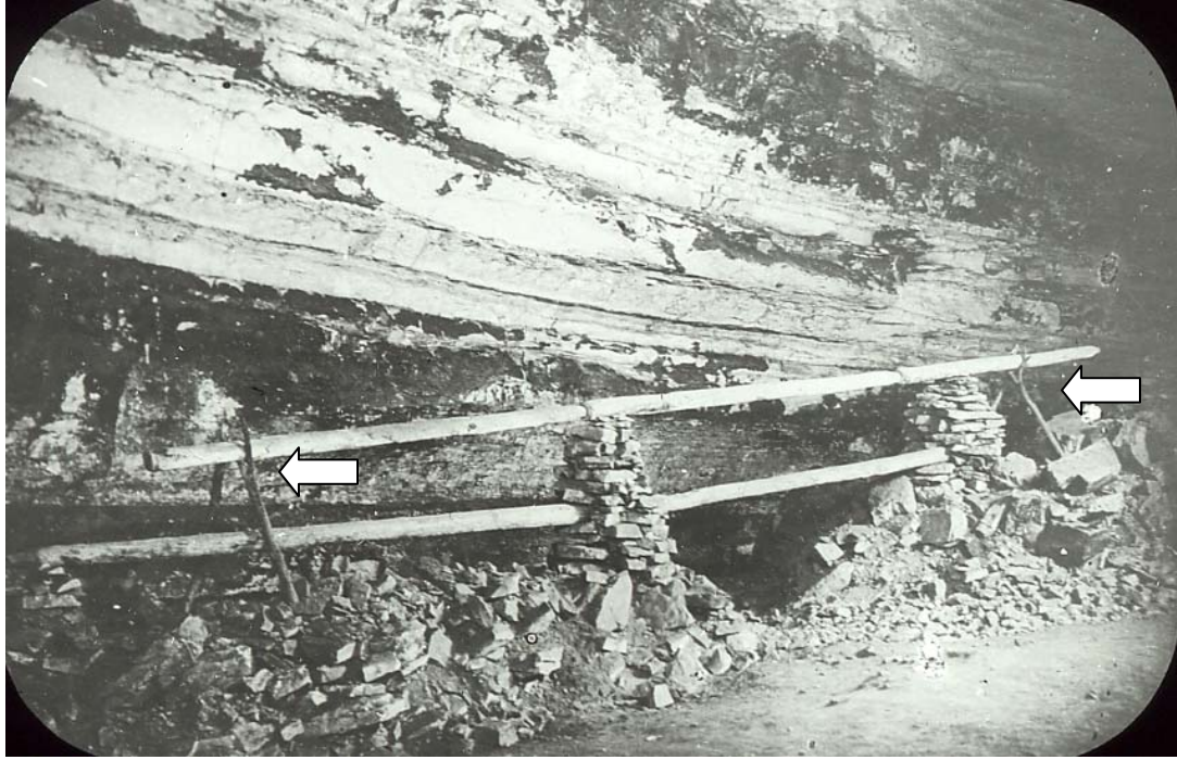
Figure 30. Examples of Y-shaped “flagpoles” used in construction of the water transport system in Mammoth Cave. (Mammoth Cave Series, Mammoth Cave, Kentucky. Old Entrance. Sections of original wooden pipe in position as they were used in securing salt peter; one line brings fresh water in, the other line carries water, loaded with salt peter, out. slide, The Jesse Earl Hyde Collection, Case Western Reserve University [CWRU] Department of Geological Sciences, Cleveland, Ohio).
