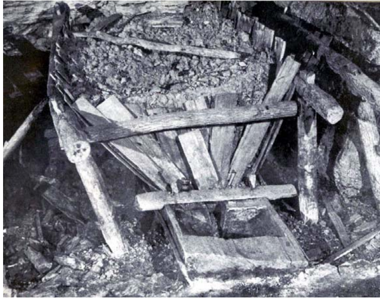
Figure 1. Example of a V-shaped vat type in Calfkiller Saltpeter Cave, Tennessee (Matthews 1971: 6).
