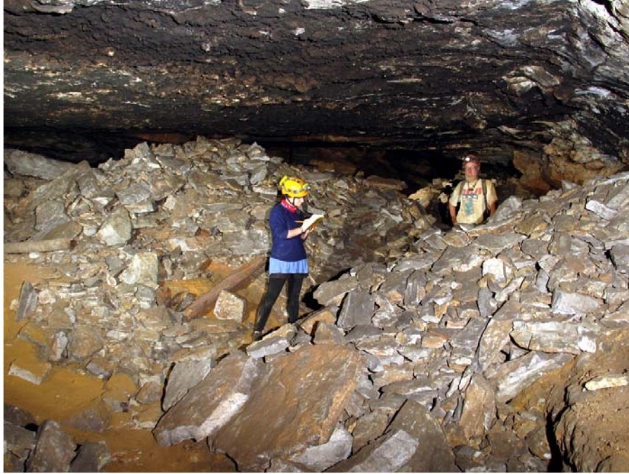
Figure 23. Ceiling breakdown moved by the saltpeter miners in Area C of Cagle Saltpetre Cave. Photo by Alan Cressler.
